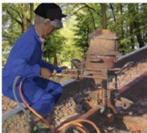
Figure 3.11 Thermit process for joining railway tracks
