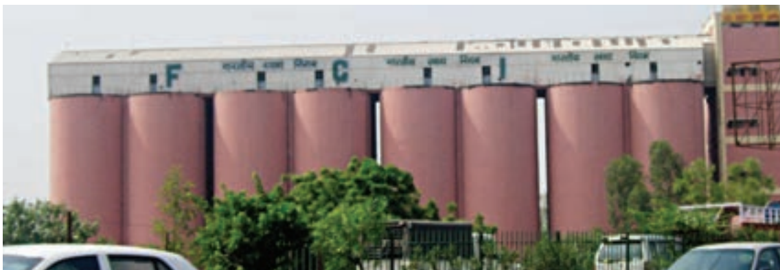
Fig. 1.10 (a) : Silos for storage of grains
